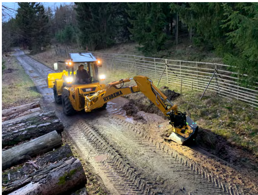
The pulling of drainage ditches on the side of the forest path is very easy with the view to the excavator arm
