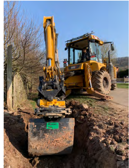
HYDREMA's multi-purpose backhoe loader replaces a 10 ton mobile excavator ditching
