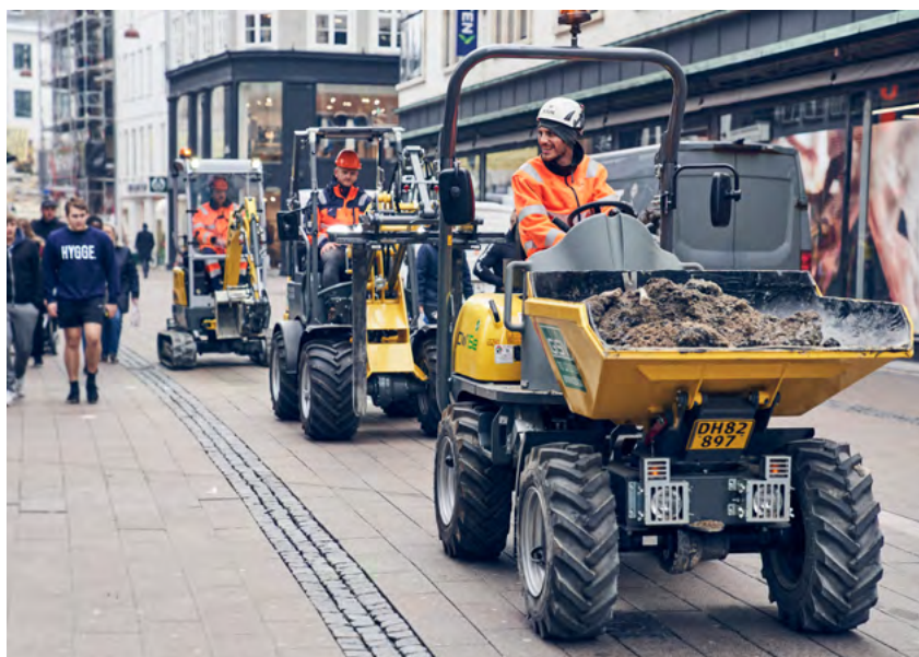
Electric and battery machines in action, Copenhagen
