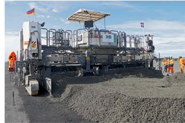
At Keflavik Air Base, the Wirtgen SP 62i delivered precise single-layer concrete paving with a width of 7.62 m (25 ft) and a thickness of between 41 cm (16 in) and 45 cm (18 in).
