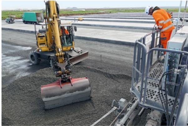
The concrete was placed in front of the SP 62i slipform paver by an excavator and then evenly distributed with the machine's spreader plow.
