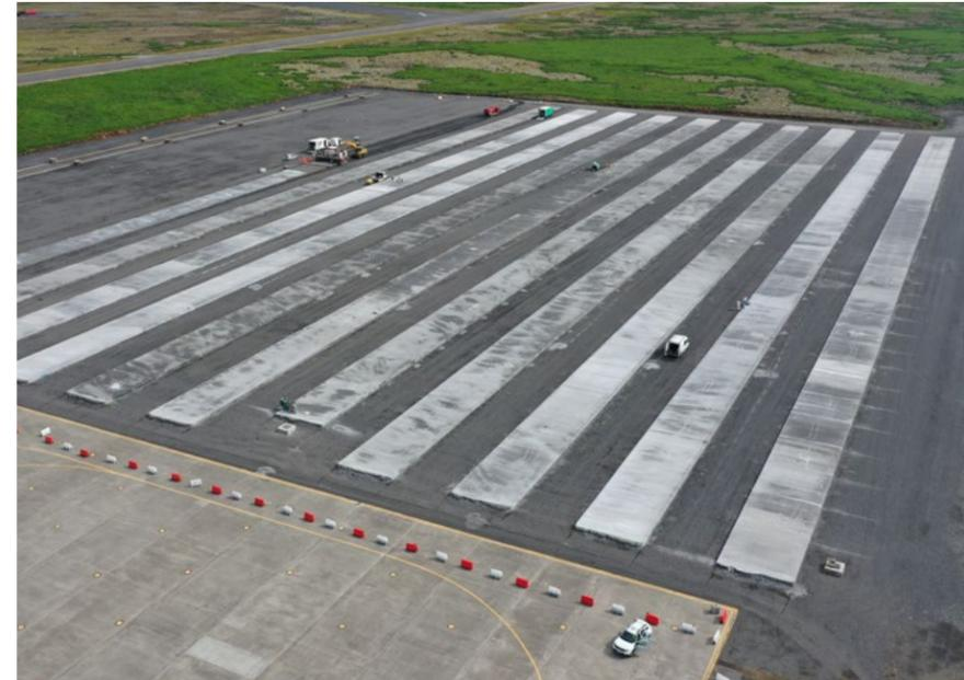
The extension of the parking apron is realized in the form of 31 separate strips connected to one another by tie bars inserted along their sides.
