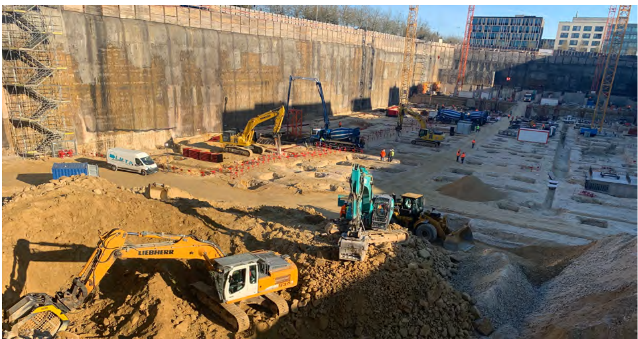
Limestone recycling - BF120 crusher bucket and MB-S18 screening bucket used by Kobelco SK 350 and Liebherr 934
