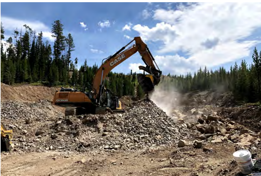
BF120.4 crusher bucket mounted on Case CX350D crawler excavator
